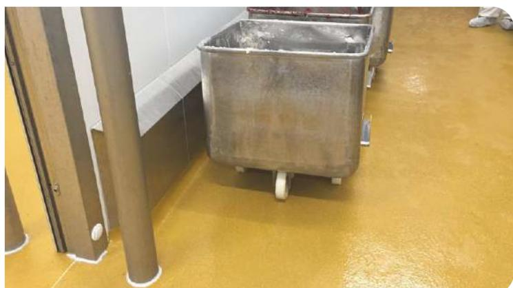
PolySto prefabricated **ICS40RB** stainless steel kerb with concrete core with a resin floor applied into the rebate.
